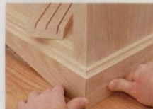
Install the base skirt
